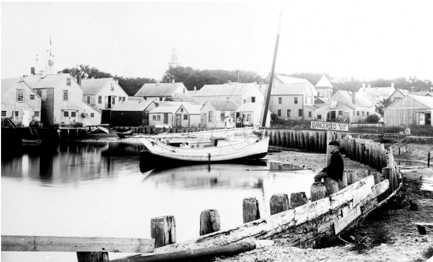
Figure 18.—Leaks between the planks of catboats were caulked on beaches at low tide, Nantucket, Mass., about 1920. Photograph courtesy of Nantucket Historical Society.
