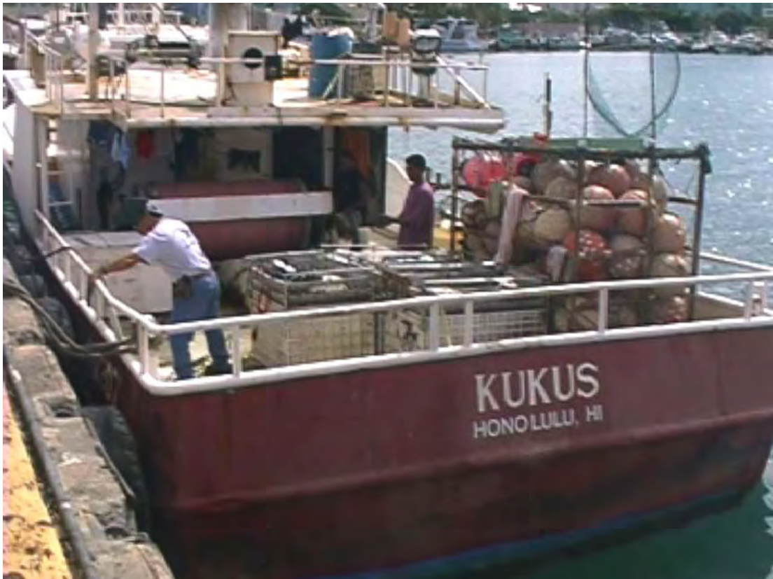
Fig. 25. Main line shooter mount being installed on the port side of the F/V Kukus.
