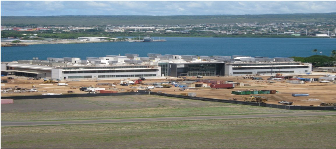
Figure 4.—NOAA Inouye Regional Center at Ford Island under construction.
